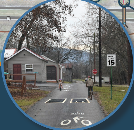
Sharrow and speed cushions on Locust Alley bike boulevard
